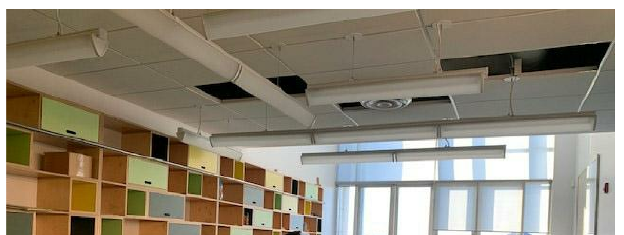
2 - PROGRAM ROOM CEILING
